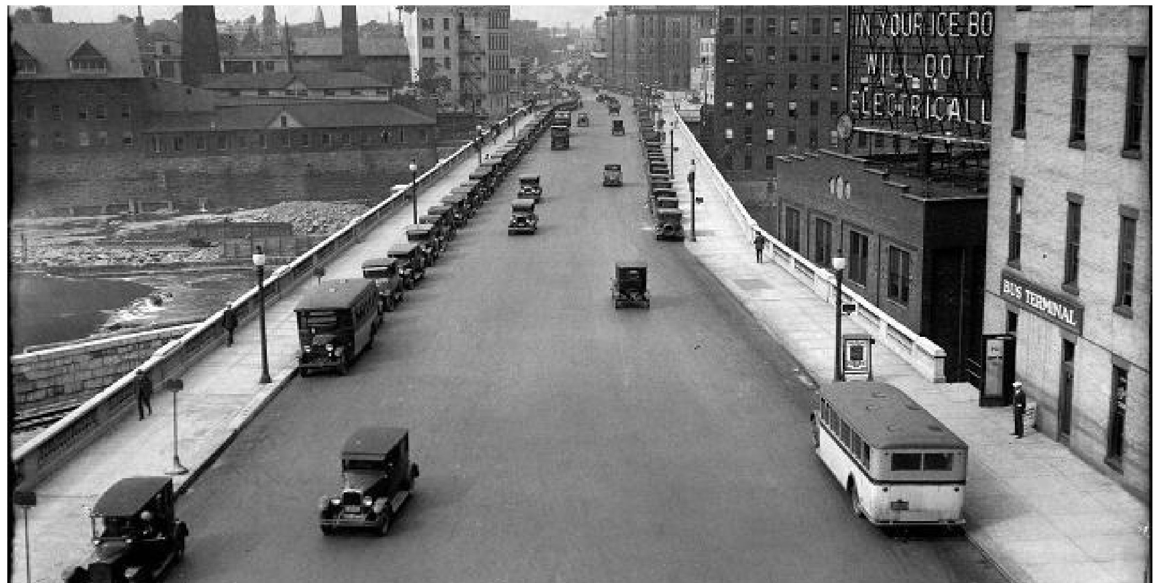
Broad Street Bridge (1925)
