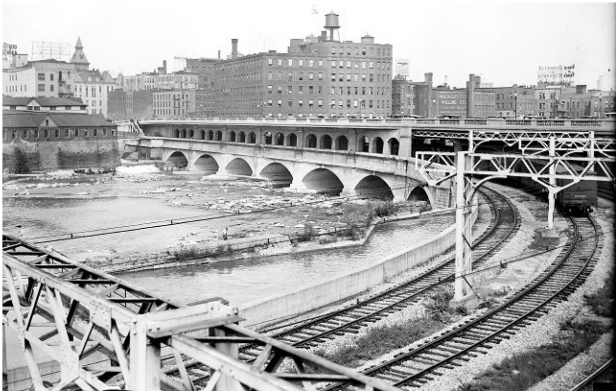
Figure 3.3 Historic photograph of the aqueduct adapted for subway use and Broad Street Bridge roadway
