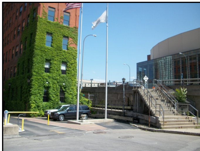
Currently the deck of the Broad Street Bridge runs along the second story of the building occupied by Thomson Reuters but this will be removed during the aqueduct restoration
