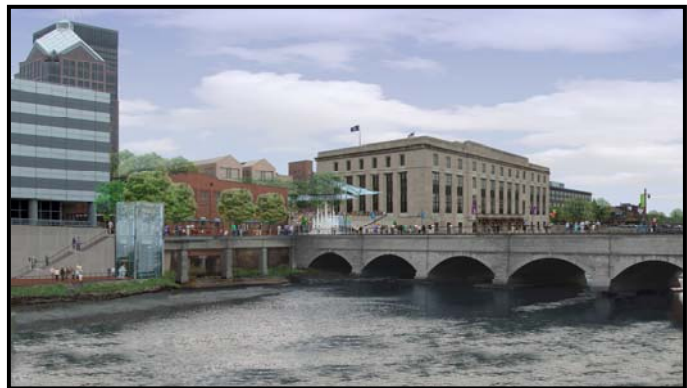
Phase 1 restores the aqueduct to its 1842 appearance and opens up viewsheds along the Genesee River
