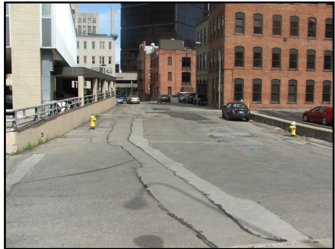
Existing condition of Aqueduct Street looking north to Main Street
