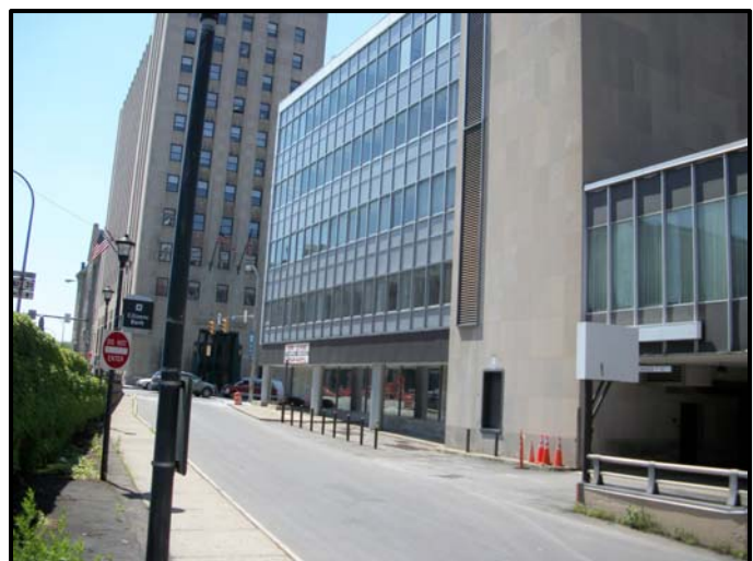
Currently no green space exists in front of 44 Exchange Boulevard which is planned for adaptive reuse as market rate apartments
