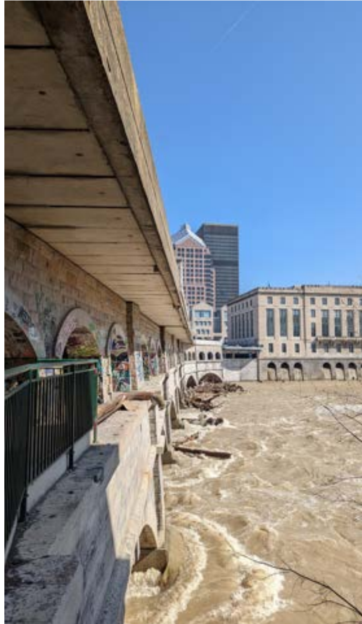
Aqueduct from War Memorial
